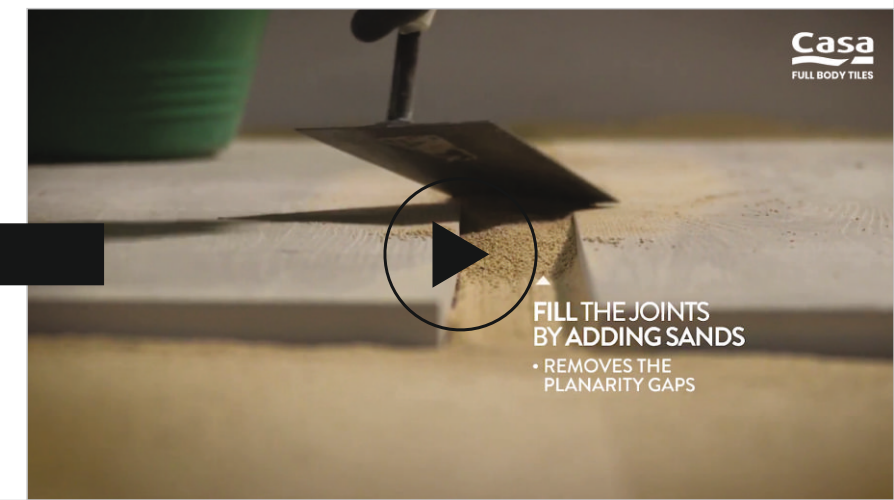
LAYING ON SAND
