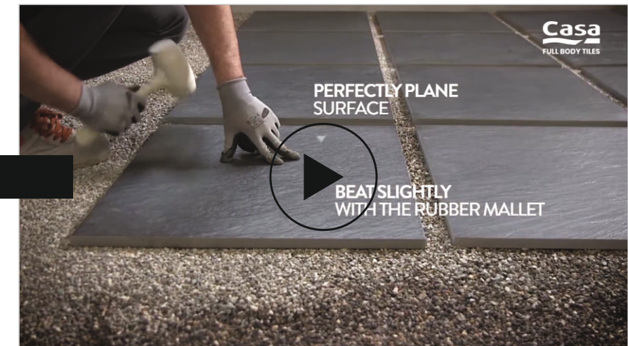
LAYING ON GRAVEL
