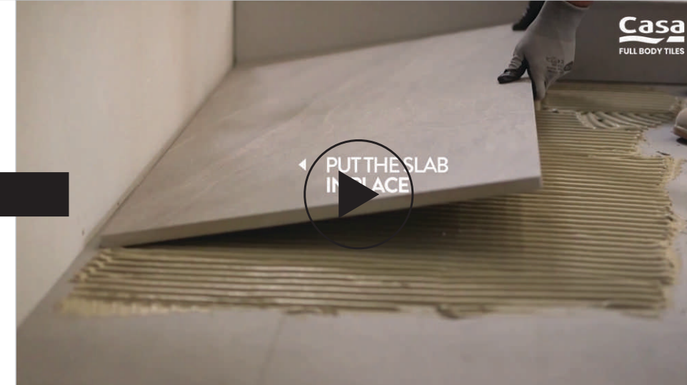
LAYING ON SCREED
