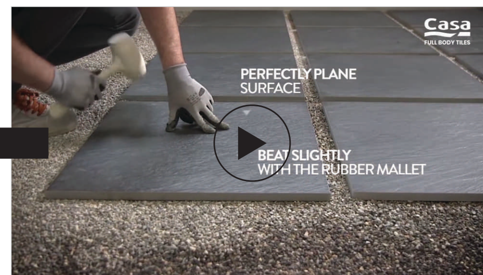
LAYING ON GRAVEL
