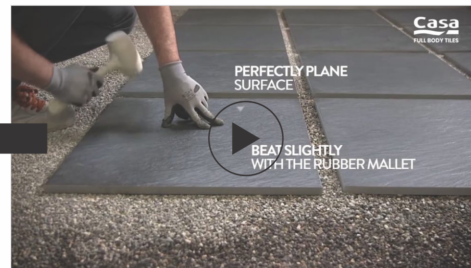
LAYING ON GRAVEL
