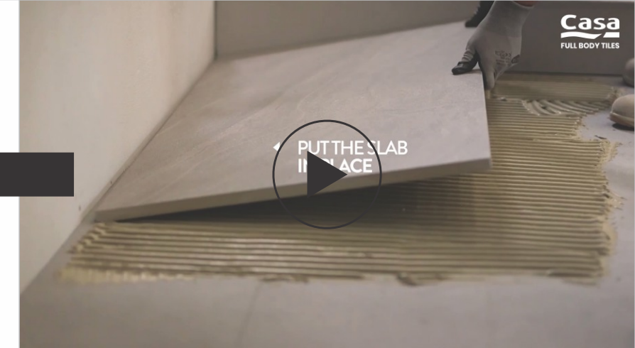
LAYING ON SCREED
