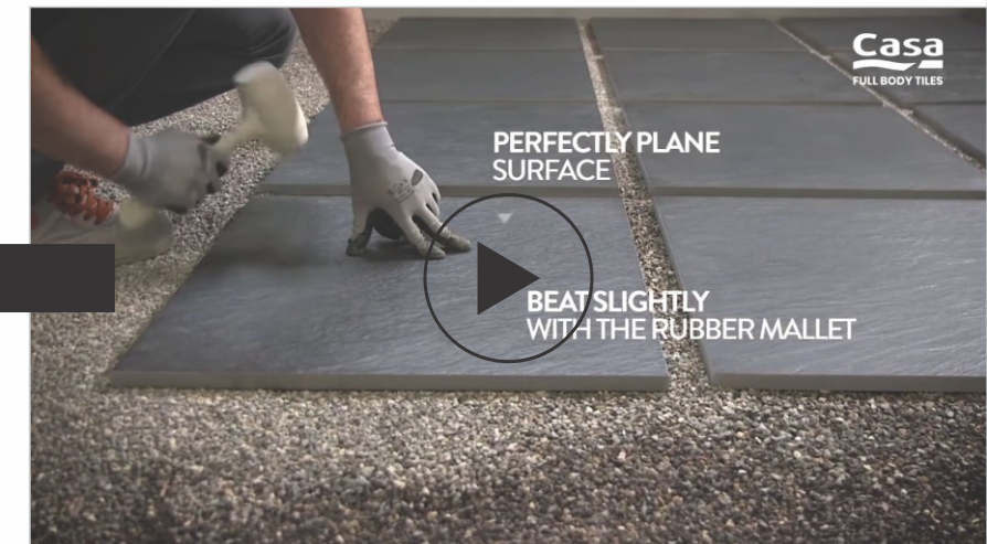
LAYING ON GRAVEL
